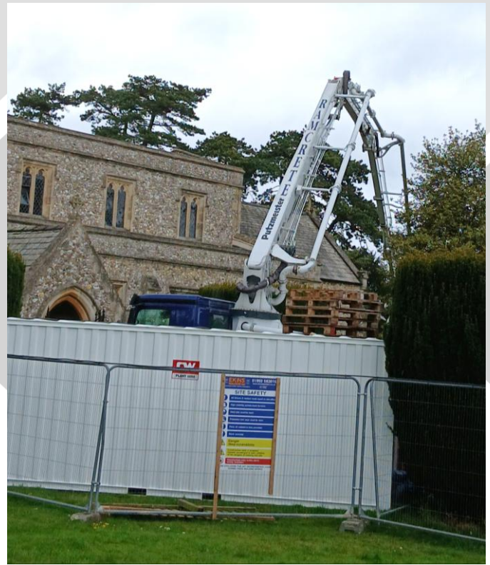
Concrete was pumped over the church roof to provide foundations
