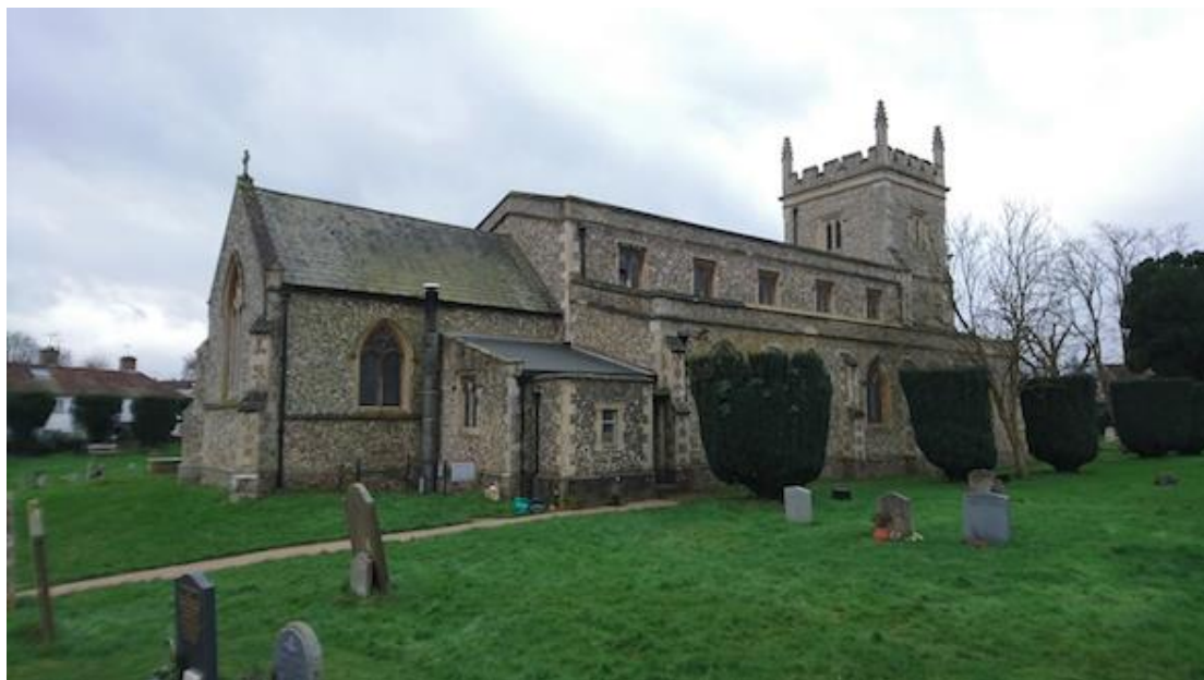
North Elevation: From the NE looking over to the location for the extension
