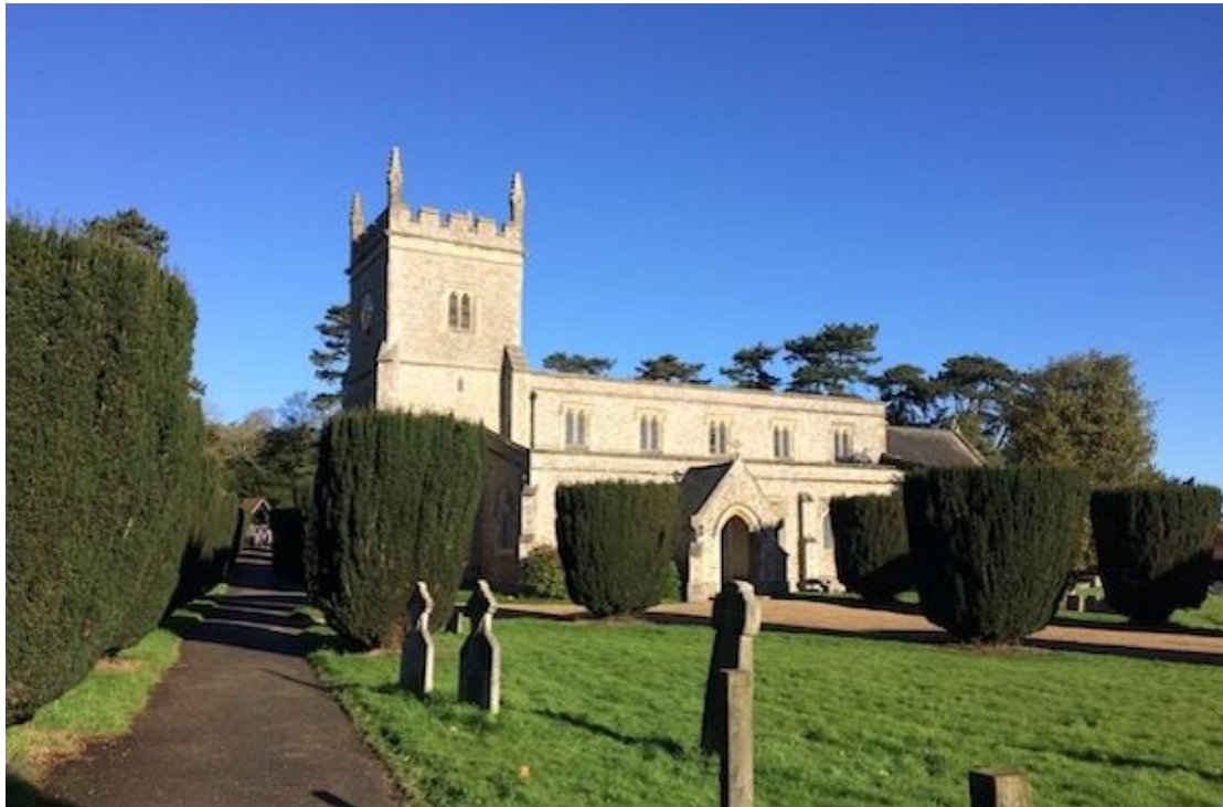
South elevation: viewed from the main path.
