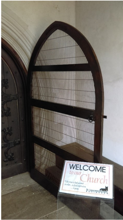
Restoration of benches and bird door in the south porch
